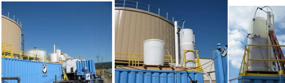
DEFERUM 24 Pilot Set up
